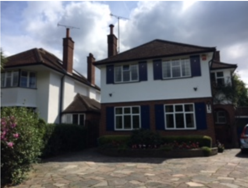
Southern side of the application property and adjoining neighbour to the south (no. 43)
